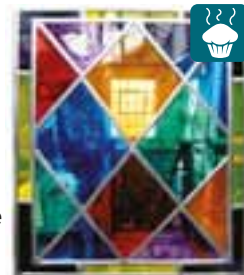
Glass window with self-adhesive lead and painted with Hatolite
