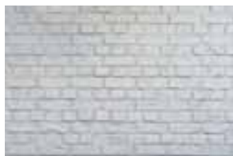
Brickwall English Bond Brickwork
